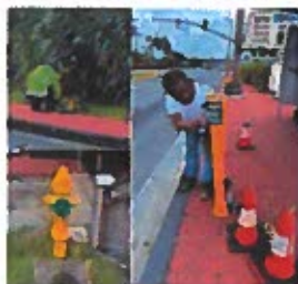
Repainting of Fire Hydrants & Bollards
